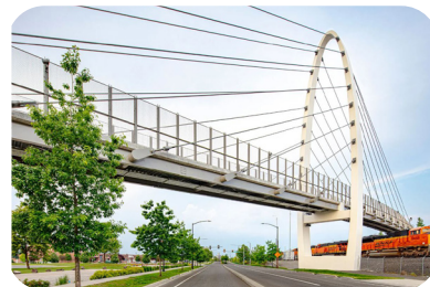
University Gateway Bridge Pullman, WA Length- 450'
